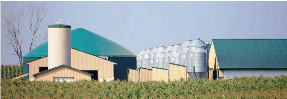
Anaerobic digester that processes swine waste and heifer waste at Feerlings Hillside Swine Farm in Overisel, Michigan; Source: FPPC
