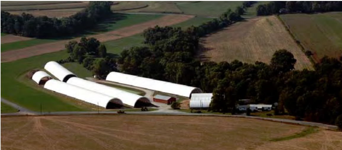
Composting facility at Oregon Dairy; Source: http://blogs.edf.org/oregondairyorganics/
